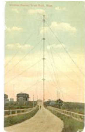
Brant Rock transmitter
