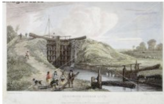
Double lock, Thames and Severn Canal, 1814
