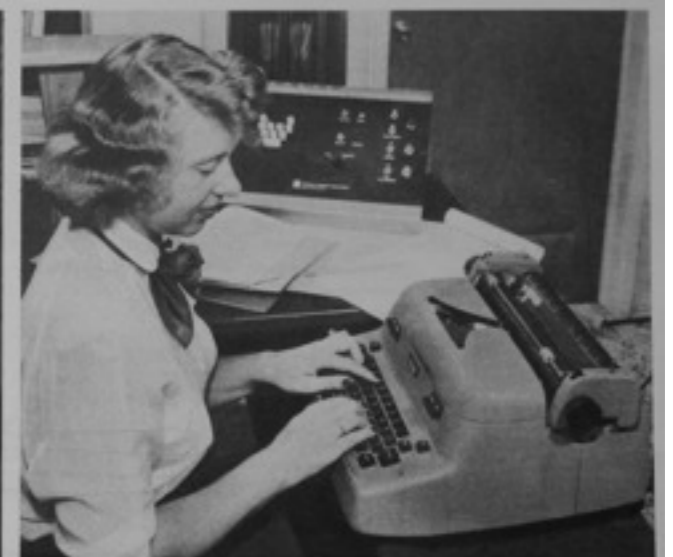
The keyboard and electric typewriter, above, are linked to CADAC, latest approach to an automatic general computer—a 195-tube machine with magnetic-drum memory (see page 117) tucked away in a closet. Computer Research Corp. will offer it to business.
