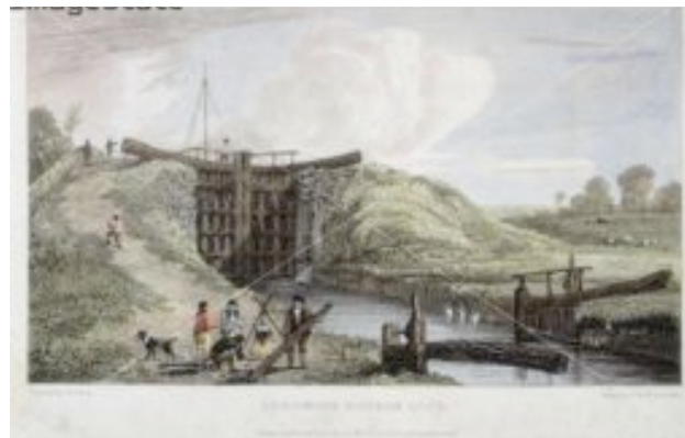
Double lock, Thames and Severn Canal, 1814
